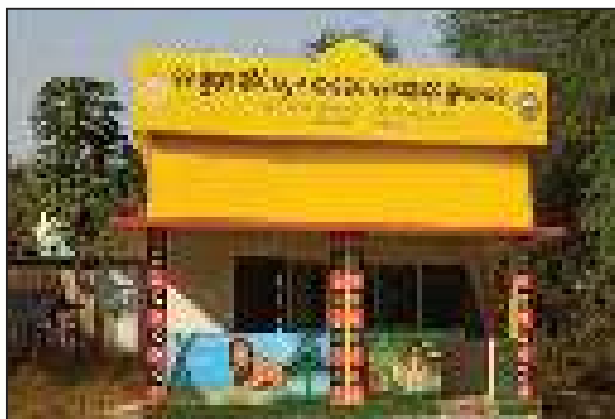
Junani VSS building built under OFSDP-II in Subarnapur DMU
