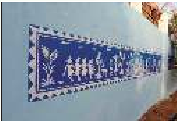
Maintenance and Beautification of existing boundary wall
