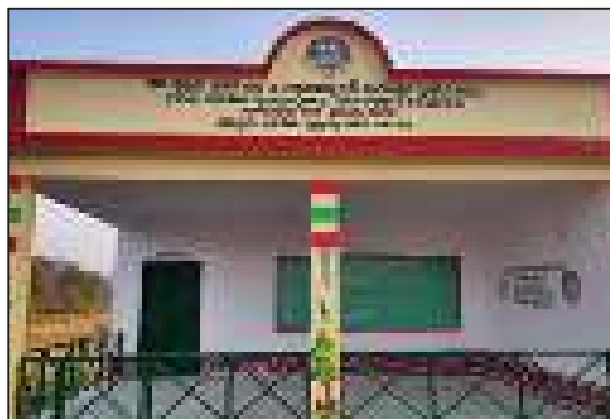
Sarapanka VSS building built under OFSDP-II in Ghumusur (South) DMU
