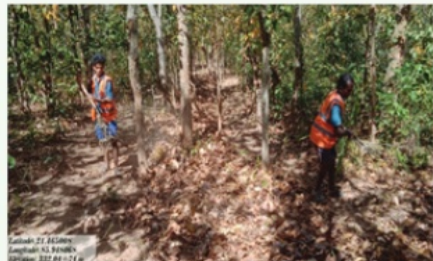
Fire Line creation work at Atei ANR Site, KeonjharForest Division
