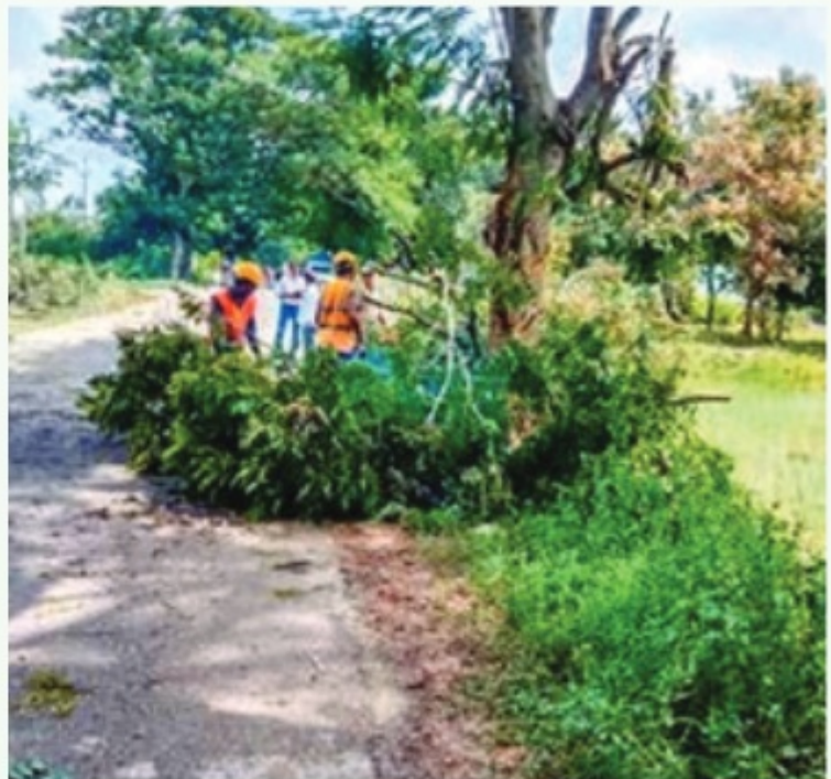
Roadside tree clearance work
