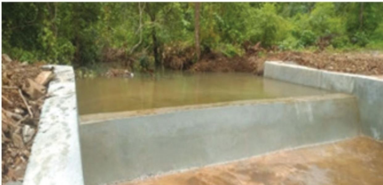
Check Dam constructed after analysing the Drone Data
