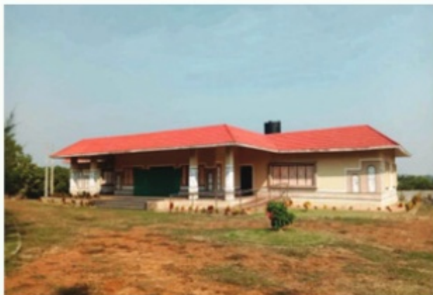
Repairing of OTDC Hall at Ansupa
