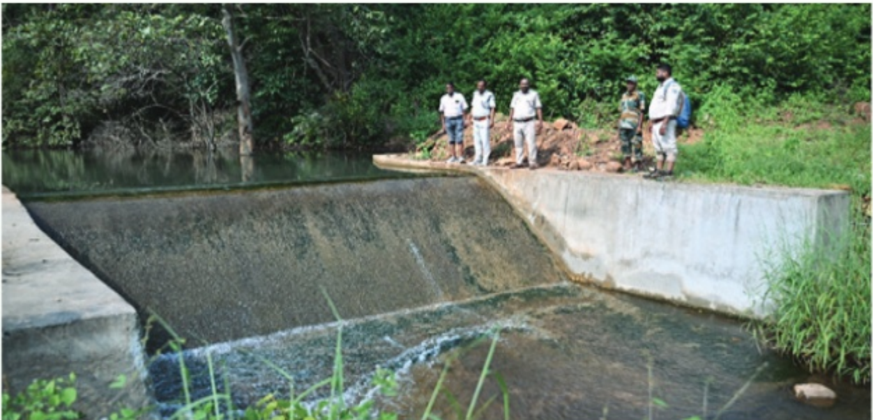
Check Dam @ Angul Division
