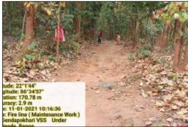
Fireline work Pithabata FMU, Baripada
