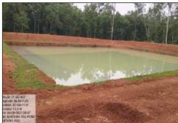
ROWHS at Bartana VSS, Betnoti, Baripada
