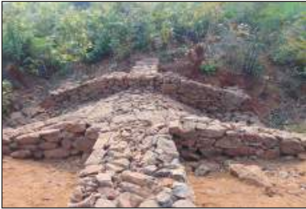
Construction of LBCD at Karunapali VSS under Boudh FMU
