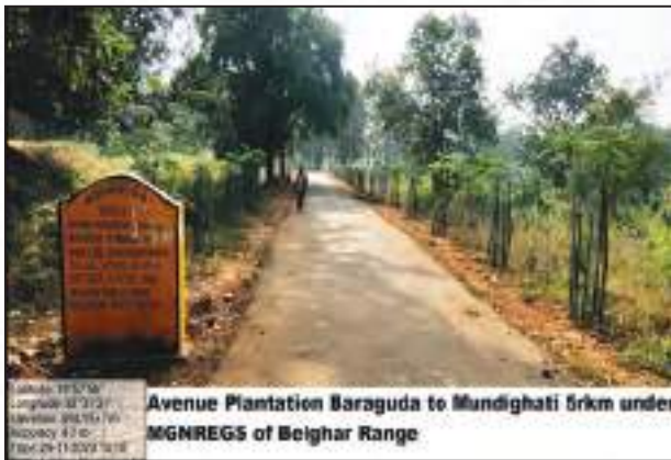
Avenue plantation under MGNREGS, Balliguda Forest Division
