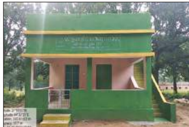
VSS building of Goudapada VSS under Sole FMU, Bonai Forest Division
