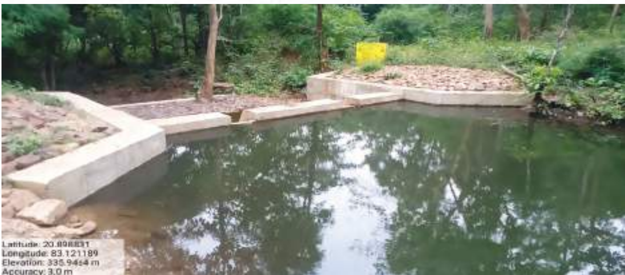
Check Dam under MGNREGS, Bargarh Forest Division
