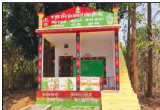
VSS Building of Gundibira, Suroda under Ghumusur South Division
