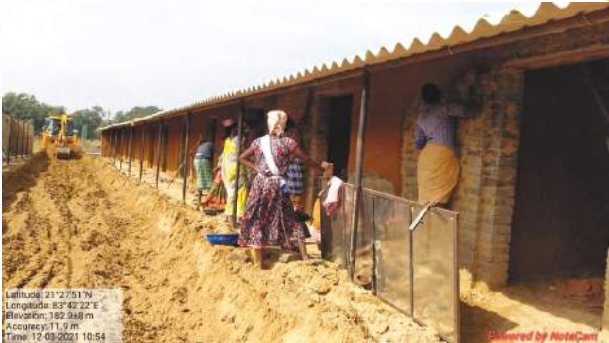
Construction work of temporary shed of Lambipali relocated village
