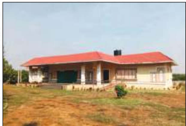
Repairing of OTDC Hall at Ansupa
