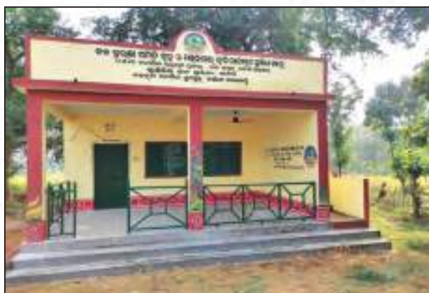
VSS Building of Kankakumar, Bagdihi under Jharsuguda Division
