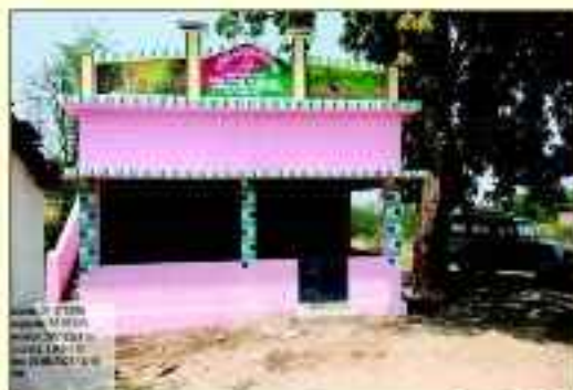
VSS building cum office at Pehpura VSS, Deogarh Division
