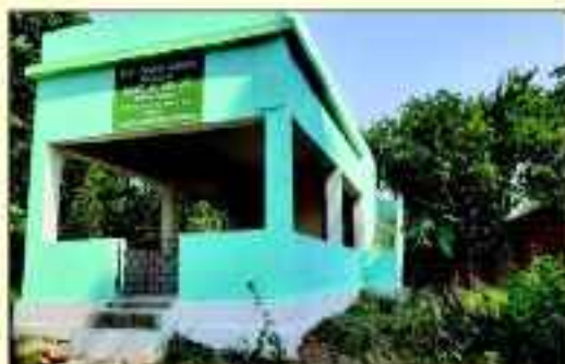
VSS Building, Palakhaman VSS, Bamra WL Division
