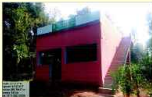
VSS office cum meeting hall at Tentuli VSS, Angul Division
