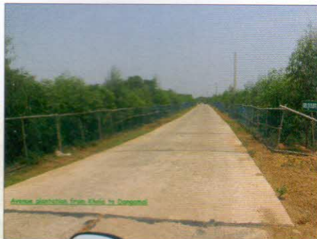
Avenue Plantation from Khola to Dangamal, Rajnagar (WL) Division
