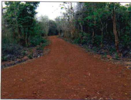
Forest Road repair, Berhampur Division
