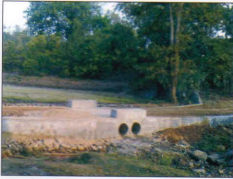
Culvert on Forest Road in Nabarangpur Division
