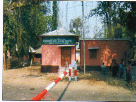
Forest checkgate strengthened at Karatapata in Angul Division
