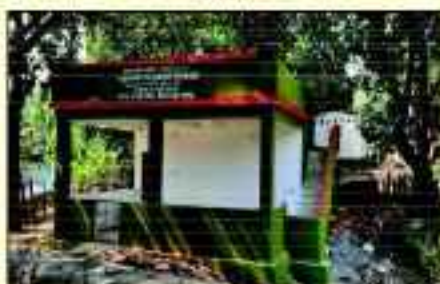
VSS building, Mayarnocher VSS, Bardo WL Division
