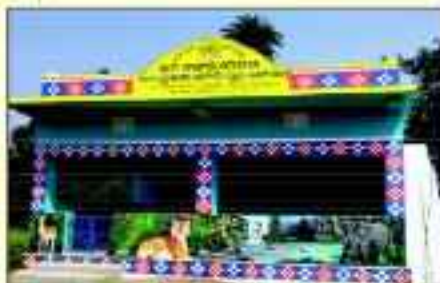
VSS office cum meeting hall at Nuzali VSS, Hubballi Division
