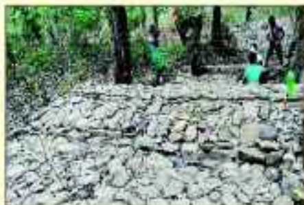
JBCD Work in Subanspur Division
