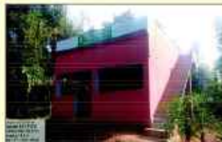
VSS office cum meeting hall at Jenua VSS, Angul Division
