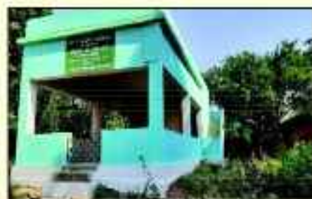
VSS building, Palakhamar VSS, Bardo WL Division
