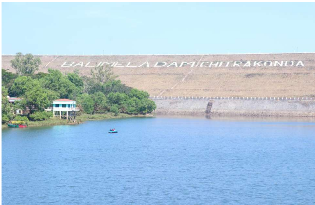
Fig. No. 1.9: Chitrakonda Dam
